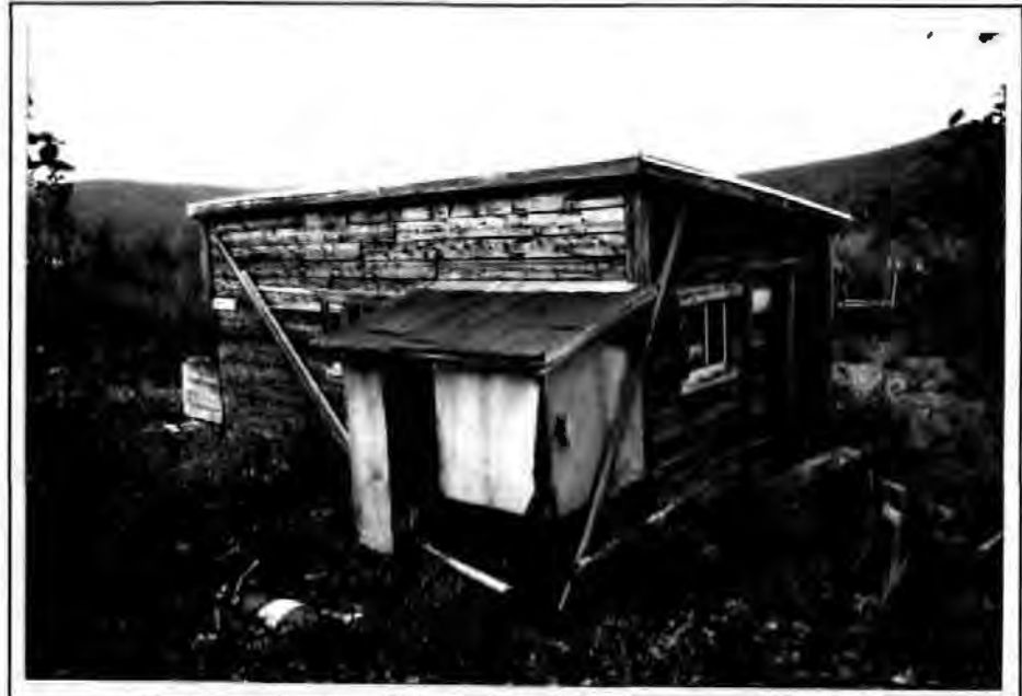
Figure 64. The Balange Carpentry Shop, 1993. The view is looking southeast.
